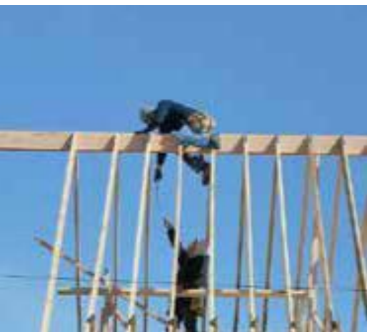
Workers constructing a home
