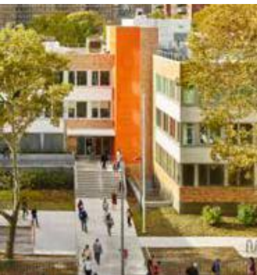
Riverside Health Center's renovation and expansion promotes health
