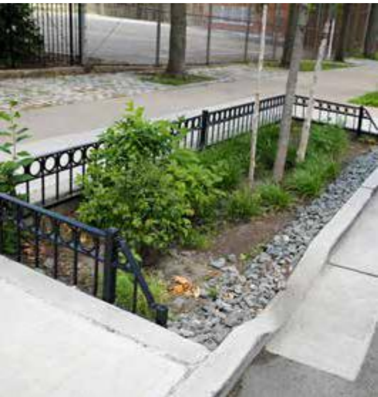
Bioswales, Hutchinson Neighborhood Demonstration Area
