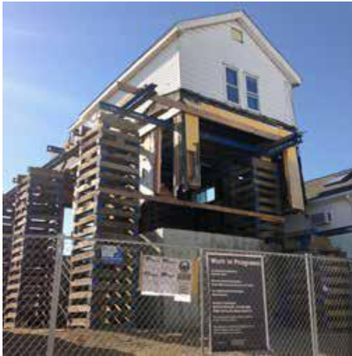
A Build it Back home elevation in Broad Channel, Queens
