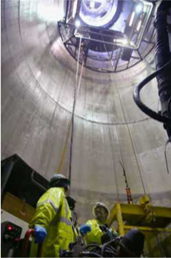
Bypass tunnel and shaft construction, Delaware Aqueduct
