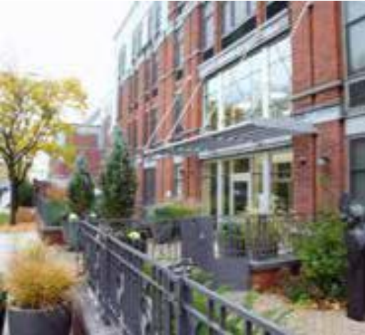
Camba Gardens Apartments in Wingate, Brooklyn
