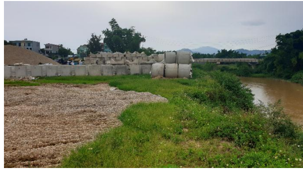
No safeguard measures prevent material dumped into Nam Rom River
